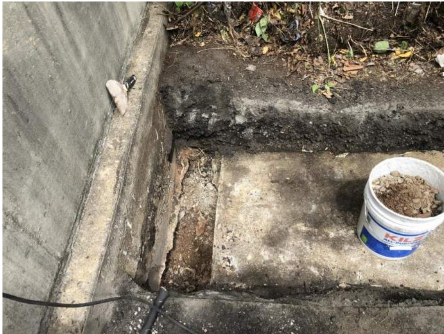
LTP-1: Concrete bridge abutment and grade beam (facing north)
