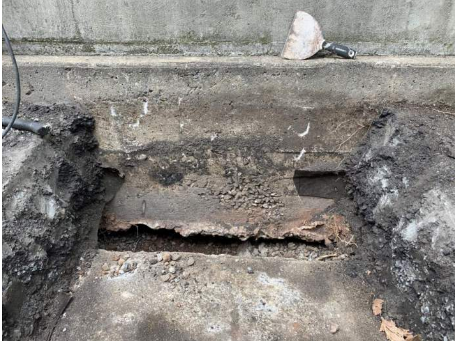
LTP-1: Concrete bridge abutment and grade beam (facing west)
